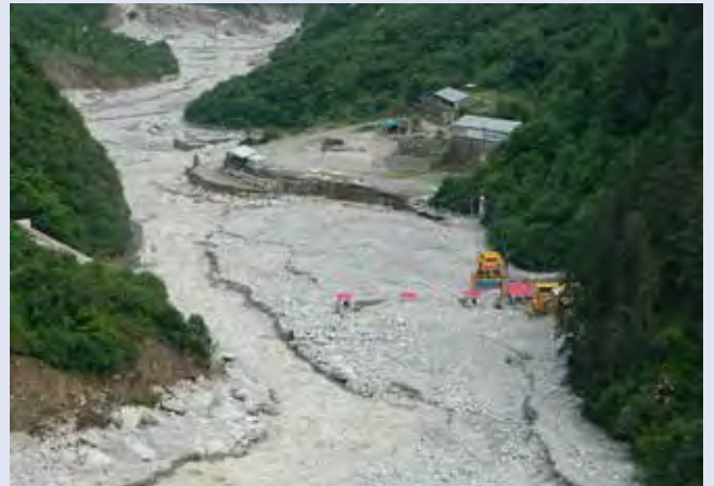
Severe flash floods swept through the Northern Indian state of Uttarakhand in 2013, destroying several hydropower projects including the Vishnuprayag Dam. Photo: Matu Jansangthan
