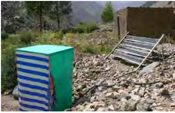
A solar water heater and shower designed by the local NGO Tajik Seeds. Photo: © Robert Middleton
