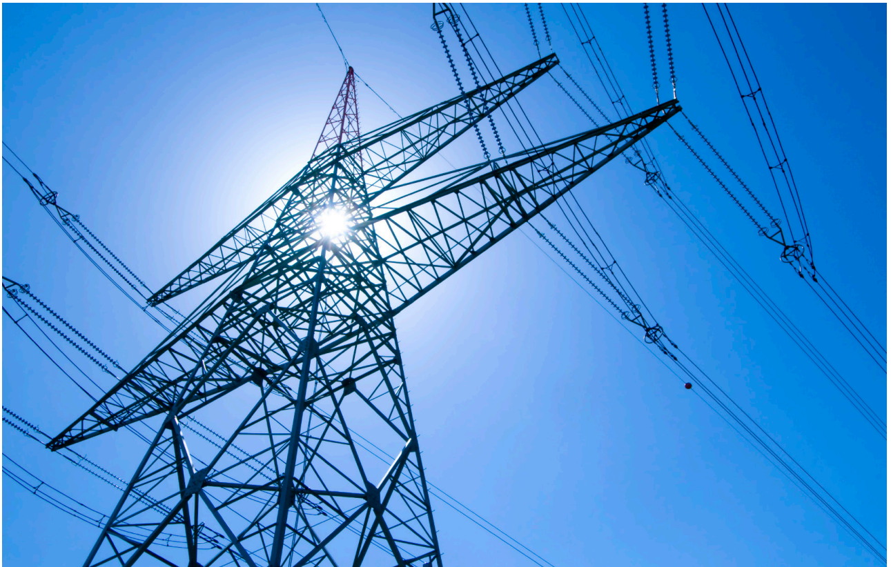
An electricity pylon. Photo courtesy of Google Images.
